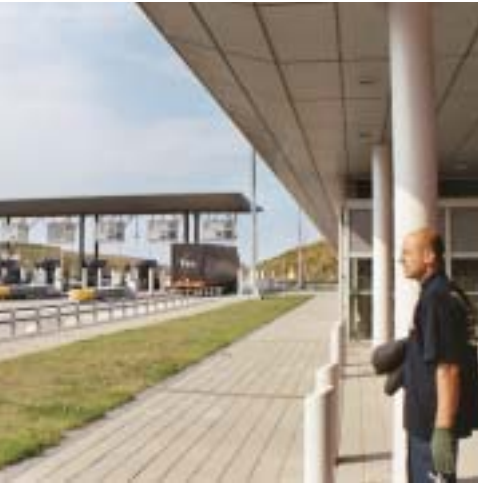
Hr. Björkmans services a toll plaza by a bridge linking Sweden and Denmark.
